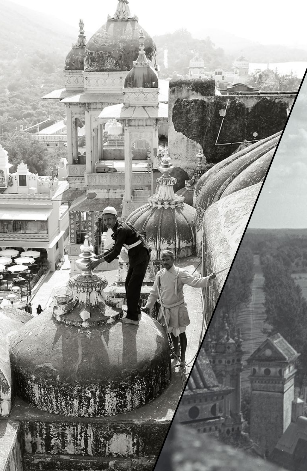
Re-installing a metal Kalasha (finial) of a Dome on Mardana Mahal, City Palace Museum of Udaipur, 2016 © Maharana of Mewar Charitable
